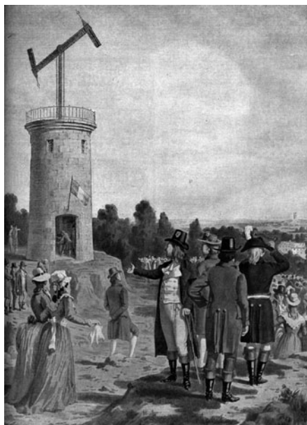
FIGURE 1.11 A semaphore telegraph tower on the first line from Paris to Lille (1794). (Leemage/Getty Image)
